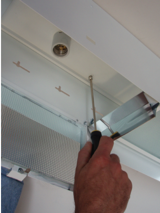
ADJUST ALL LAMP AIMING with single screw
